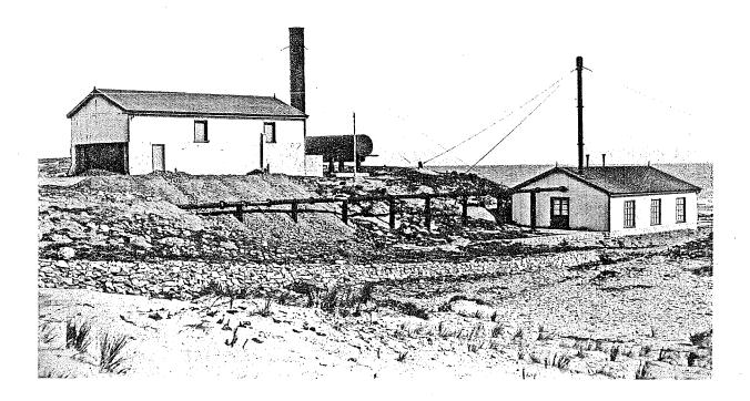
Rossiter's Point Pumping Station was erected in 1901 to pump sea water at high tide 3.6 km to Moonta Mines for use in the Cementation Works. The water was conveyed in a 23cm diameter cast iron pipe lined with wood to prevent corrosion. The original 90cm intake pipe can still be seen where it extended 200 metres into the sea.
